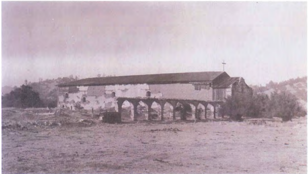
Circa 1911-1914 – Following restoration of main chapel and demolition of quadrangle wings
