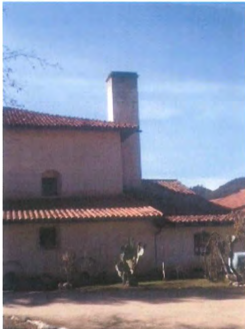
Diesel boiler chimney installed in late 1940's to be removed
