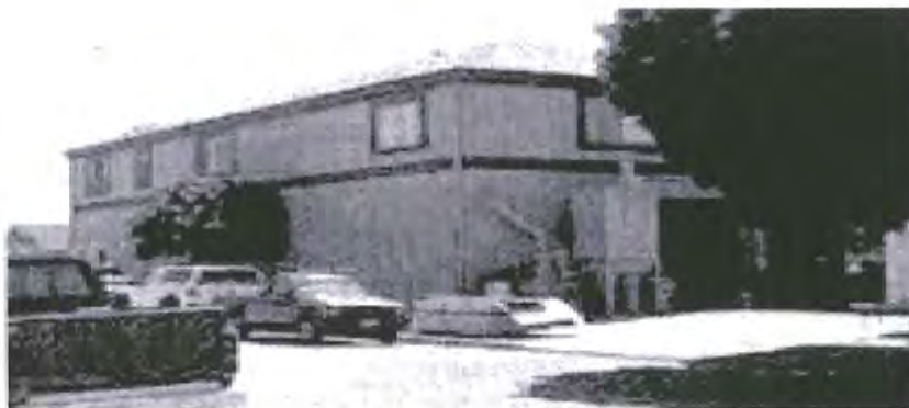
Two story Commercial Building
