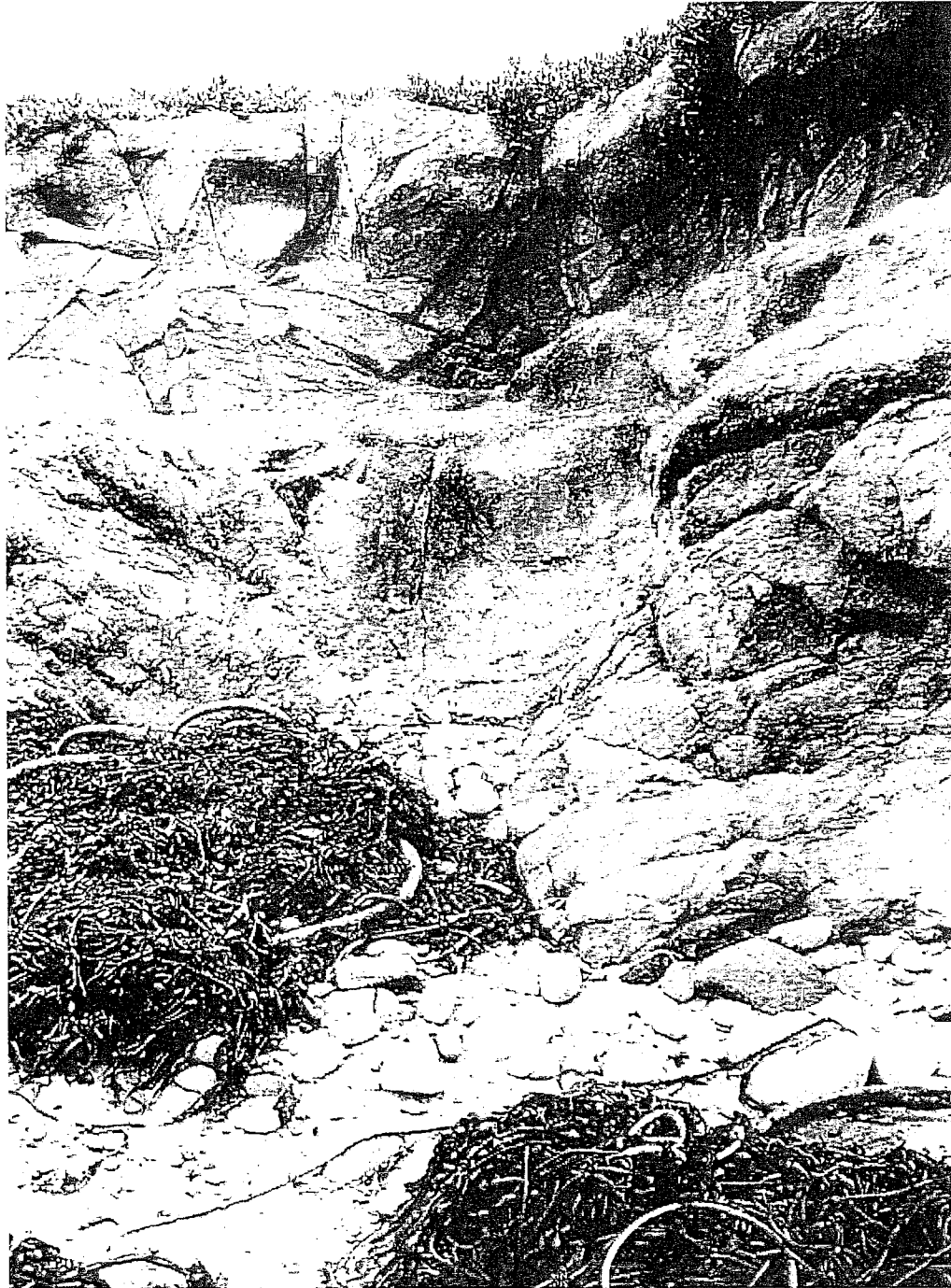
Figure 12. Short section of soil naʻi wall in Pebble Beach area , which mimics and is indistinguishable from the bluff forming granite.
