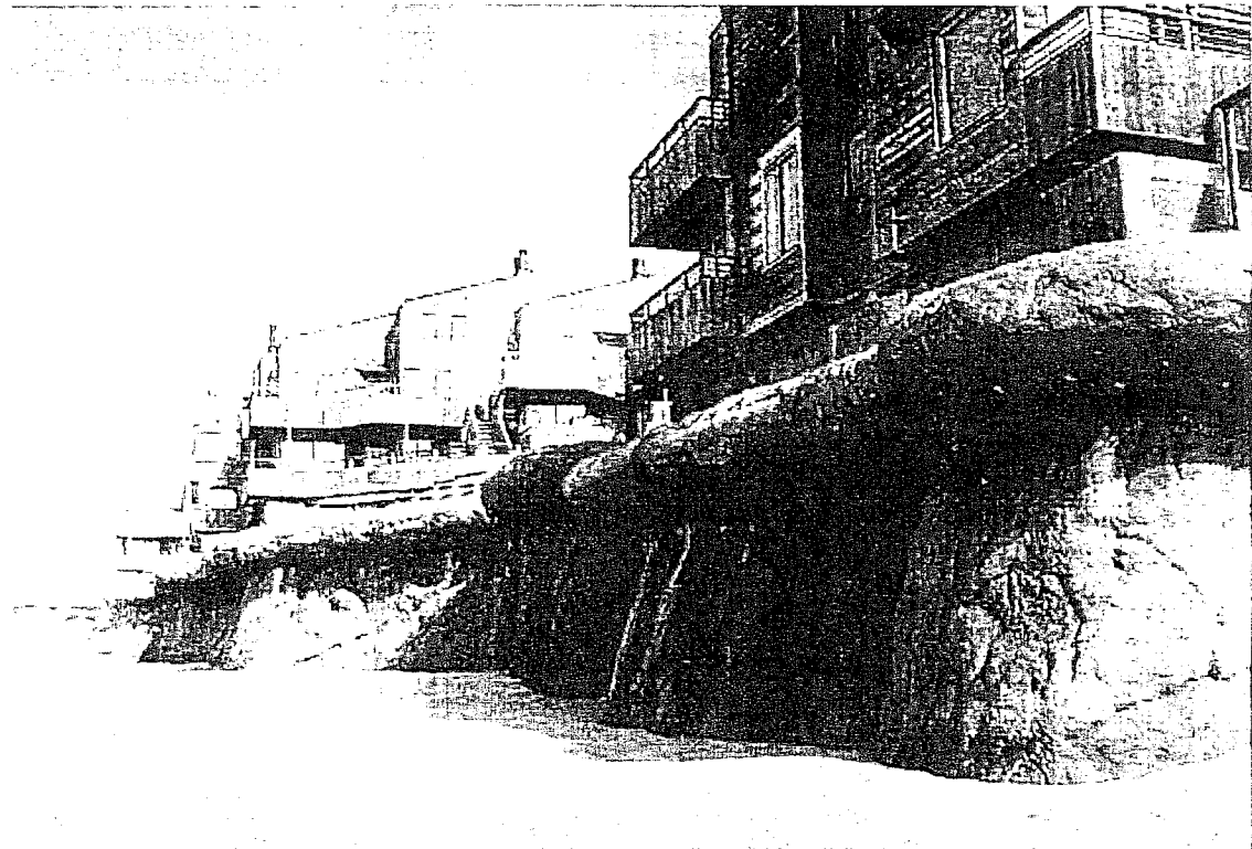
Figure 15. Concrete seawall protecting Ocean Harbor House, which blocks lateral beach access at high tides.
