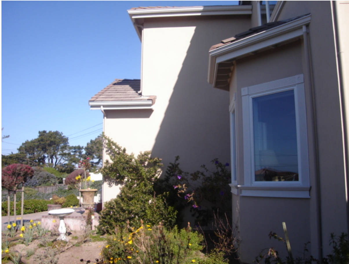
Addition area looking north
