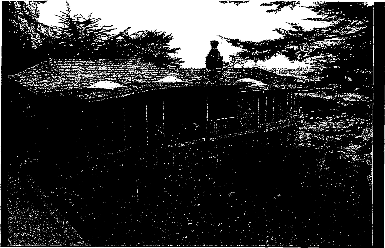
Existing Single Family Dwelling
