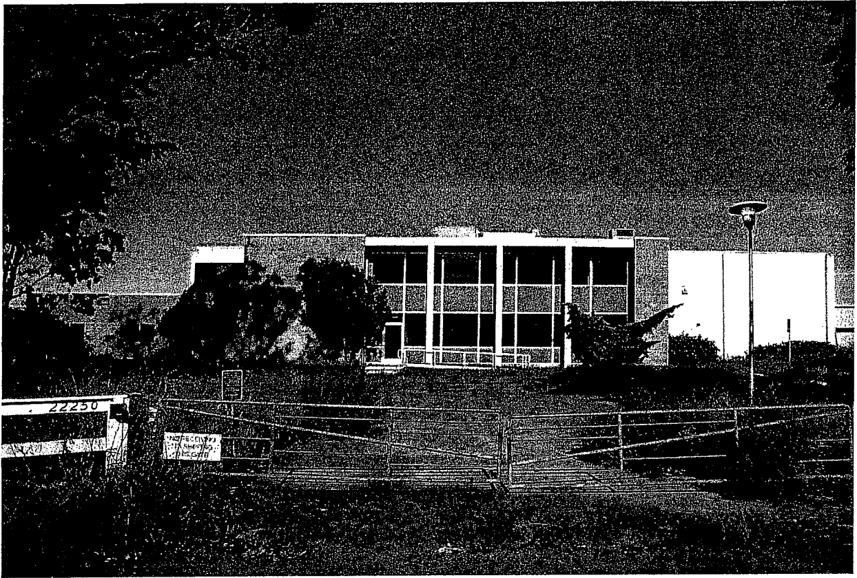
South Elevation (Front of office)
