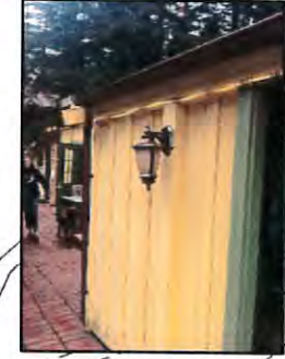
Restaurant and Retail Wall-mounted and accent rope lights
