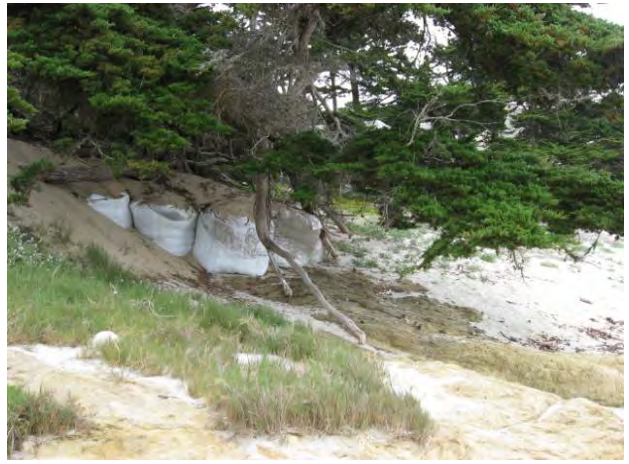
#2; View of the sand bags at the base of Cypress
