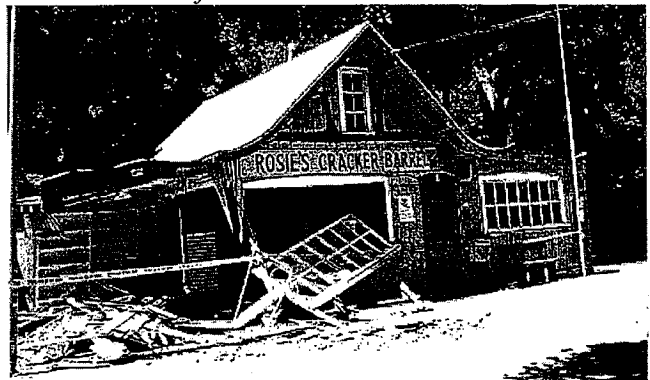
Figure 2. Damaged Sustained to Structure from Car Crash
