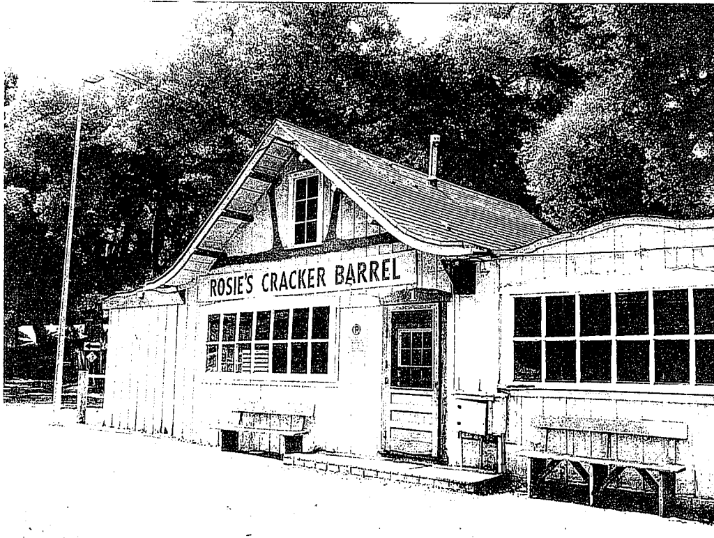
Photo #3. Looking SE at the east facing facade, June 2005.
