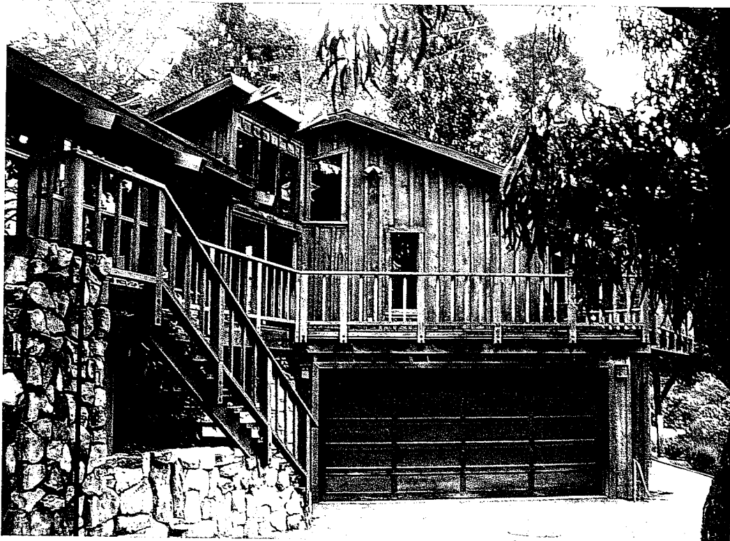
2. Looking SE at the NW facing 1983 two-story addition to the residence. July, 2008.
