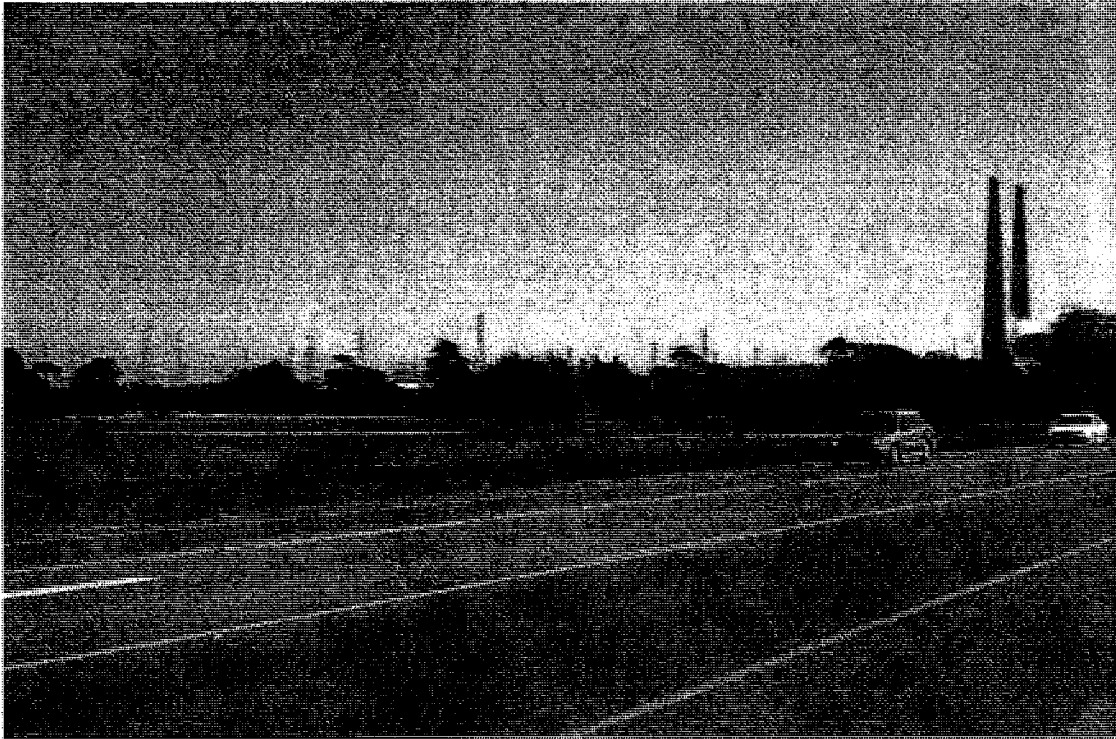
Existing view - State Route 1 looking southeast
