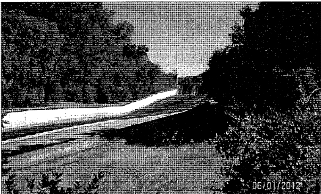
Upper stretch of spillway (Total spillway length approx. 575').
