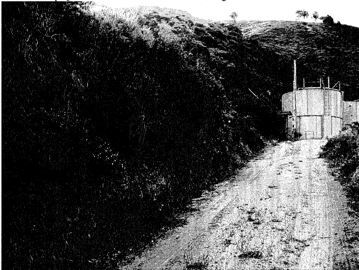
Photo 6. Post-project conditions from road location facing tank location.
