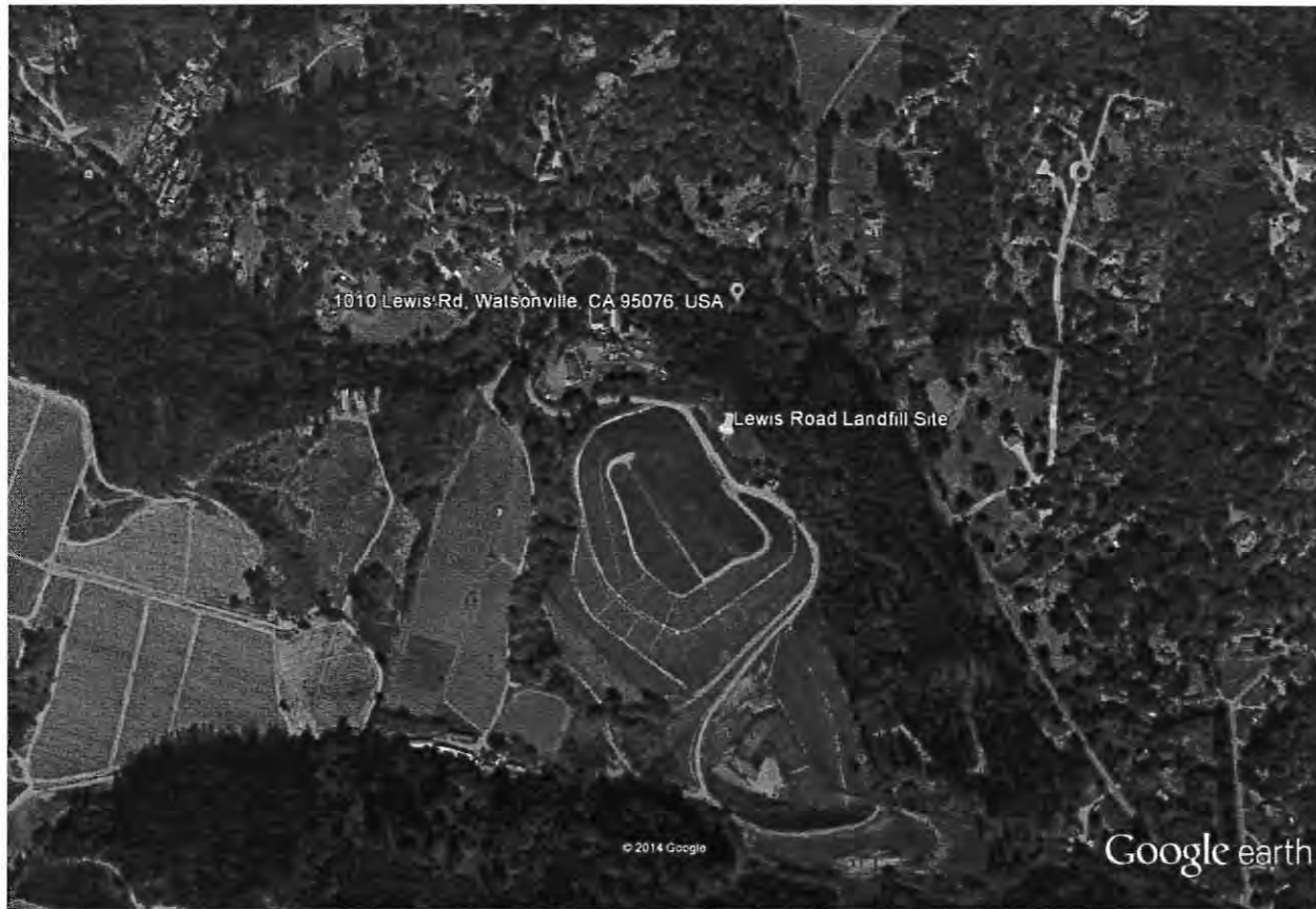
Figure 1 – Project Site Location – Aerial View
