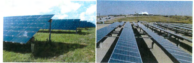
Photos 6 and 7. Examples of photovoltaic solar energy facilities
