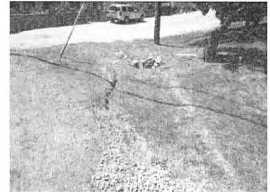
③ Unlined drainage ditch and culvert under driveway to multiple residences
