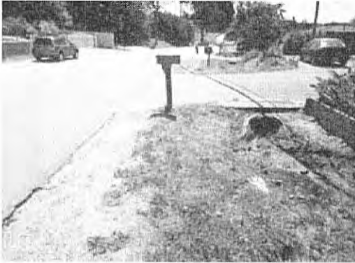
① Unlined drainage ditch parallel to Las Lomas Drive, adjacent to residential uses
