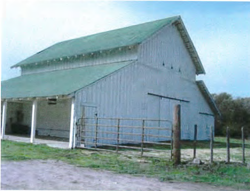
East side and covered public space
