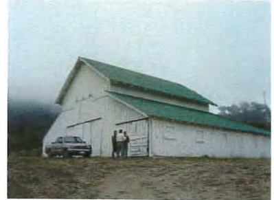
West side of the barn facing Highway 1
