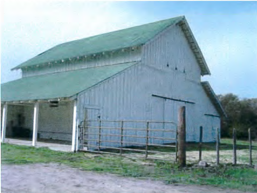
East side and covered public space
