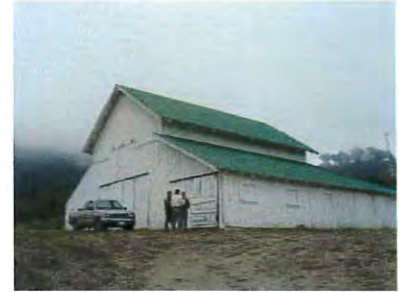
West side of the barn facing Highway 1
